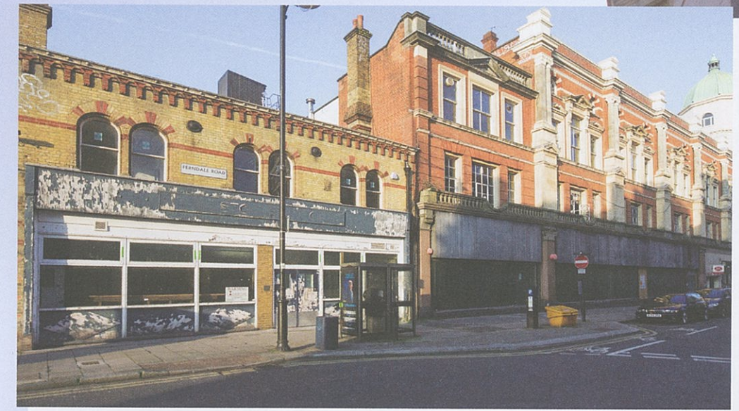
Above: Pre Construction
