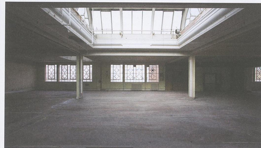
Left Page: Reception & Interior. The Department Store, Squire and Partners Above: Workspace Left: Pre Construction Photos ©James Jones
